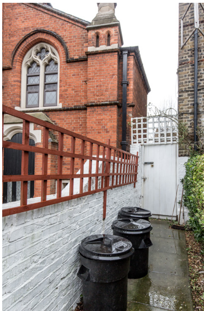
Common areas before and after upgrading 55 Croxley Road, London
