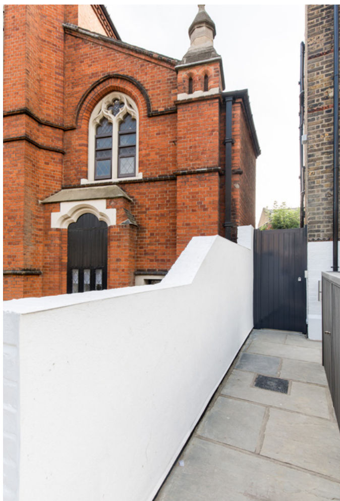
Trash bins have been replaced by proper sorting bins.
