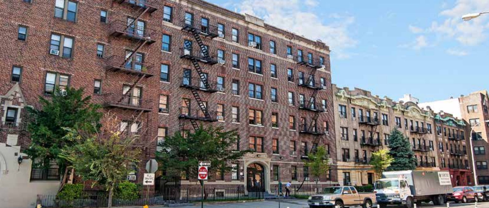
58 Linden boulevard, Brooklyn, New York, solar panels installed on the roof
