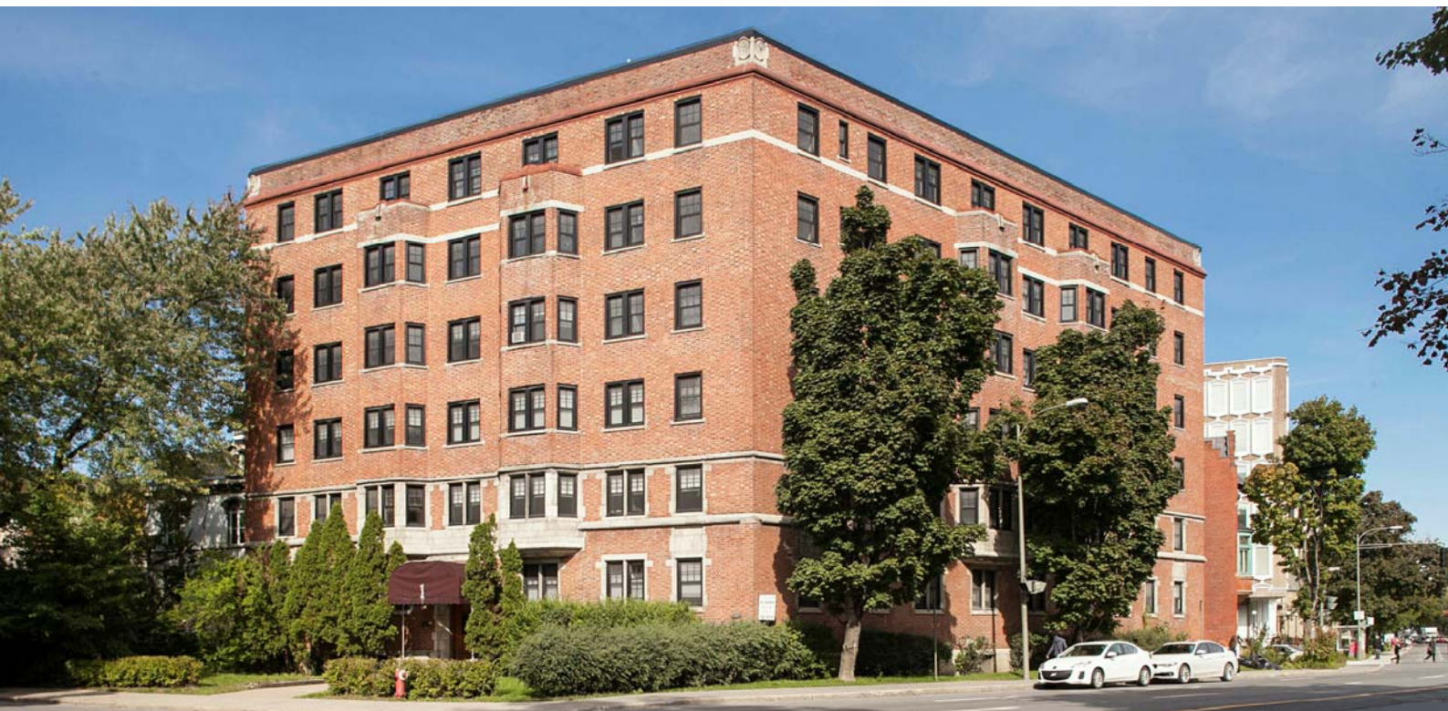
1 Rosemont avenue, Westmount, Montreal
